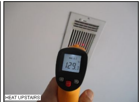
Heat tested functional - Adequate temperatures noted
