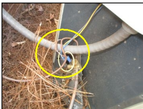
Exposed wires observed outside the AC unit - *All wiring should be placed on interior of unit
