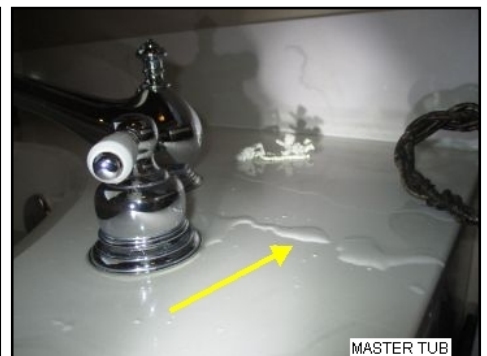
Master tub hardware leaks at base while in operation
