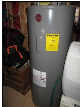
Rheem water heater - electric
