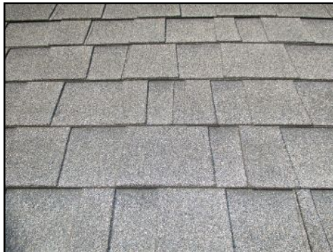
Very good granular life remaining on roofing material
