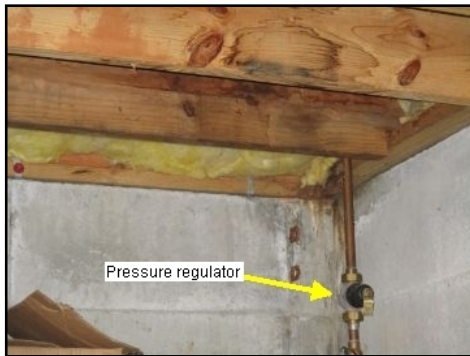
Pressure regulator noted. Basement
