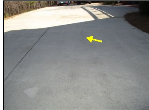
Driveway in good shape for age and wear. Minor and typical cracks. Recommend sealing to prevent expansion
