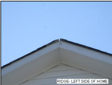
Ridge cap: deteriorated or missing shingles. Replacement of shingle required
