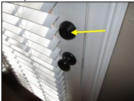
Emergency Egress Concern. Exterior door(s) have a double-sided keyed dead bolt lock set. This type of lock requires a key to unlock the door from the inside and can present an obstacle to anyone trying to evacuate the home in the event of a fire.
