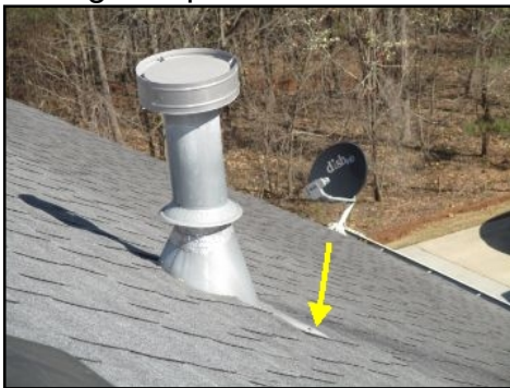
Recommend sealing all exposed nail heads
