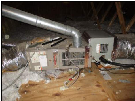
Goodman Gas furnace located in attic
