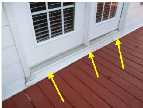
Recommend adding a kick plate to under threshold to prevent threshold damage
