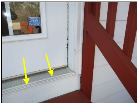
SAFETY CONCERN: The master bedroom exterior door threshold has a lip that could be a trip hazard
