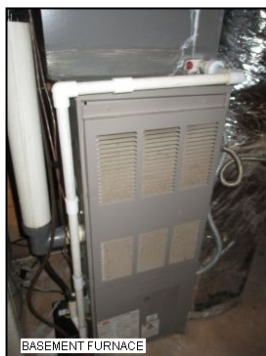
Basement furnace - Gas
