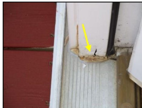
Wood deterioration observed, wood rot in trim around door jams. Suggest repairs/replacement as needed.
