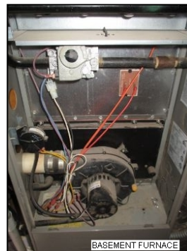
Basement furnace enclosure is clean for age of unit - Minor rust and scale
