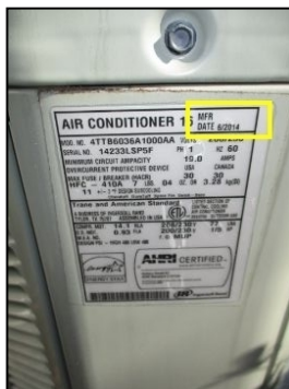
AC data plate , Brand Trane , Age 2015, 3 ton unit. Note: This unit appears to be too large for the amount of conditioned space it serves
