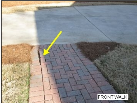
Minor settling under front brick paver walk
