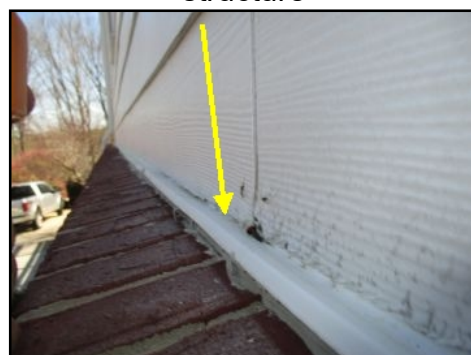
Active leaks observed at the time of inspection. Location: Under front porch and left side of structure . Source of interior basement wall leaks
