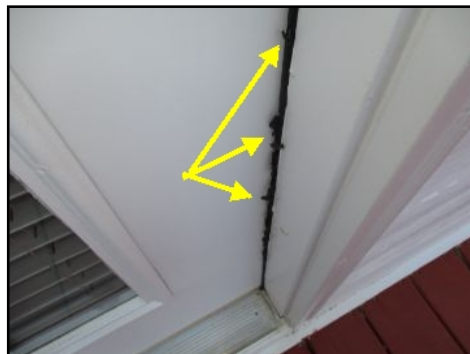
Minor repair needed- pet damage observed at several exterior door weatherstripping
