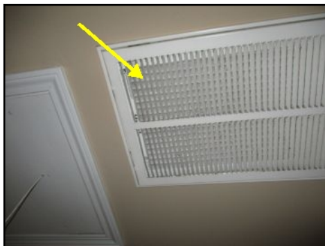
Furnace filter dirty. Needs replacement. 14x20x1
