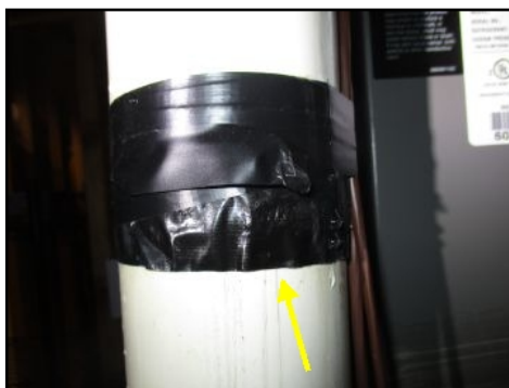
**VENTING OBSERVATIONS** Vent pipe PVC in basemen is leaking. Nonprofessional repair observed
