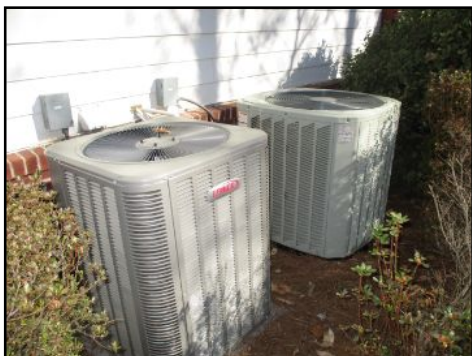
Exterior units not level. This can affect system performance. Recommend making all units level
